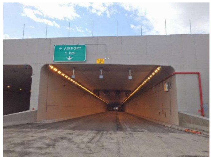
Calgary Airport Tunnel Source: Calgary City News, May 21, 2014
